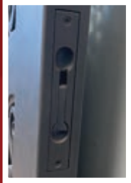
Flush bolts that pin into the door jamb
